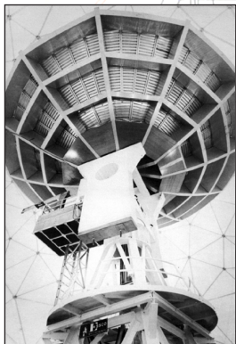
Figure 2.7 The 14 m-diameter mm-wavelength telescope at the FCRAO.
